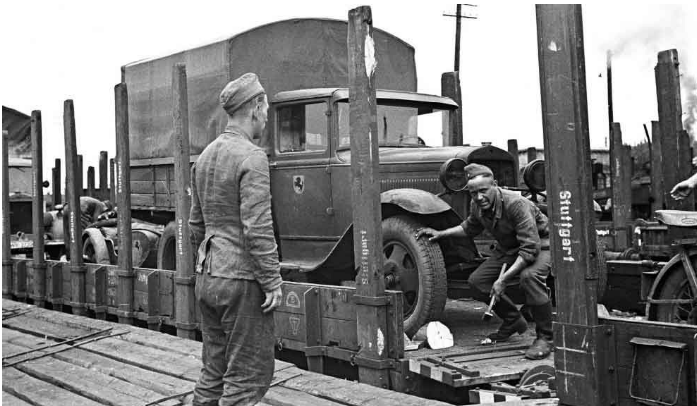
Chocking the wheels of a 1932 model Ford BB. Powered by a four-cylinder 52-hp engine, this truck was identical to the US manufactured version. The curved headlight support was straightened on the 1937 model.
