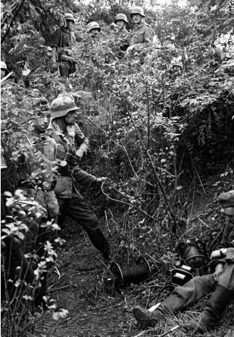
Top and above: Armed signal troops establishing telephone communication. Note the cable reels. Telephone lines of any distance were usually laid along roads and trails.
