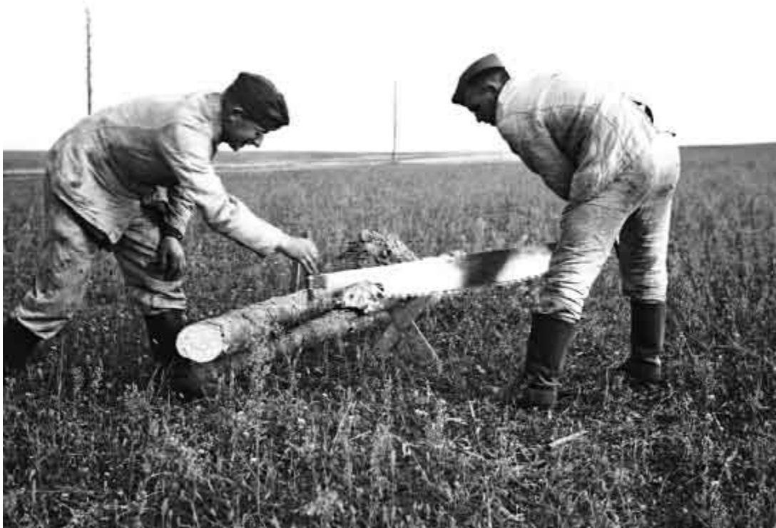
Top and above: The Drehkreuz telephone system had the practical advantage of using thin, freshly cut trees in situations where regular telephone poles were unavailable.
