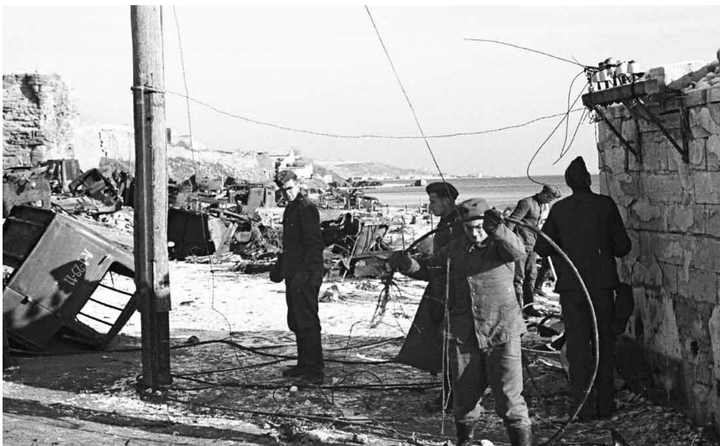
Restoring a former Soviet telephone line on the southern Crimean coast. The background resembles a Red Army 'Dunkirk' following the withdrawal of Soviet troops by sea.
