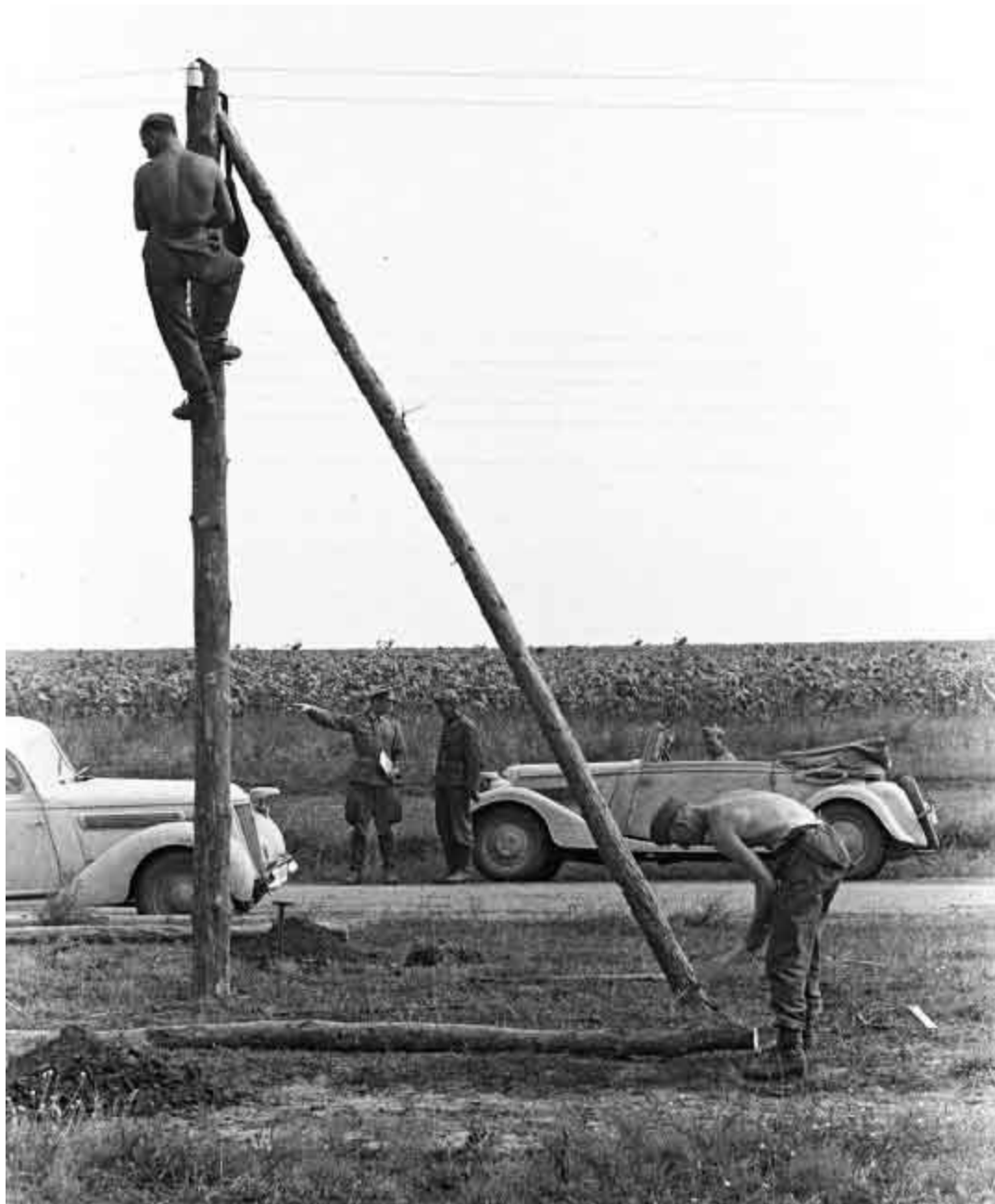
Erecting a Drehkreuz telephone line. In the background are a Wanderer 23 (on the left) and a Wanderer 240. Production of Wanderer civilian vehicles ceased in 1941 when production switched to licence-built military vehicles. Part of Auto Union, the Wanderer marque ended with the cessation of hostilities in May 1945.
