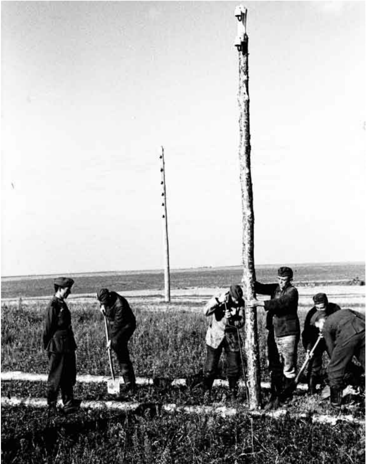
Top and above: Erecting Drehkreuz lines across the vast and featureless Ukrainian landscape. Both the Army and the Luftwaffe erected roadside telephone lines. Army lines followed the left hand side of the road (in respect to the advance) and Luftwaffe lines the right.
