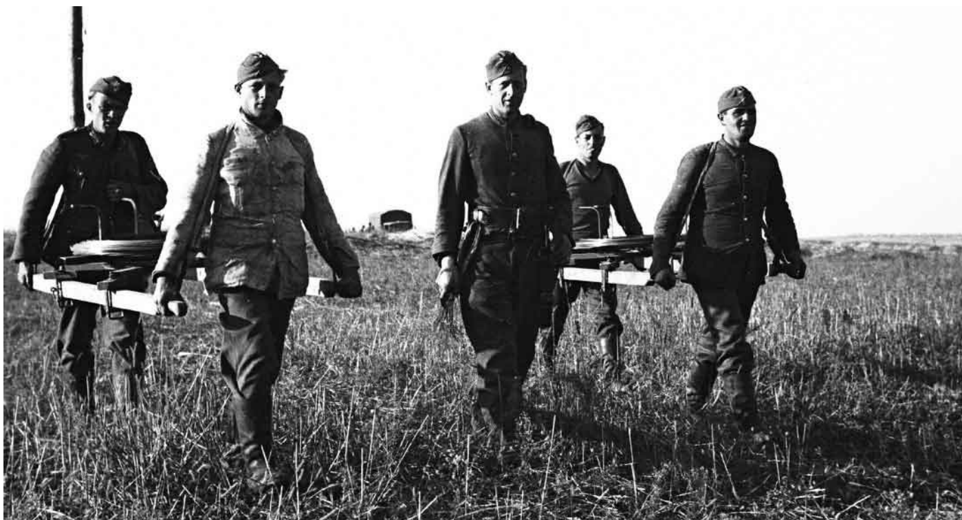
Unreeling the bare wire strung on a Drehkreuz line. Partisans generally targeted the existing poorer quality and less important Russian telephone lines, with their numerous thick iron wires, over the simpler Drehkreuz lines.
