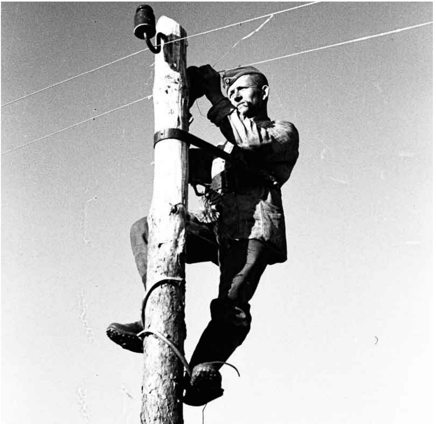
Top and above: In 1941 the Germans introduced the Drehkreuz telephone line, a simple and efficient system that significantly reduced materials and manpower. The two individual wires could carry up to fifteen telephone channels simultaneously.
