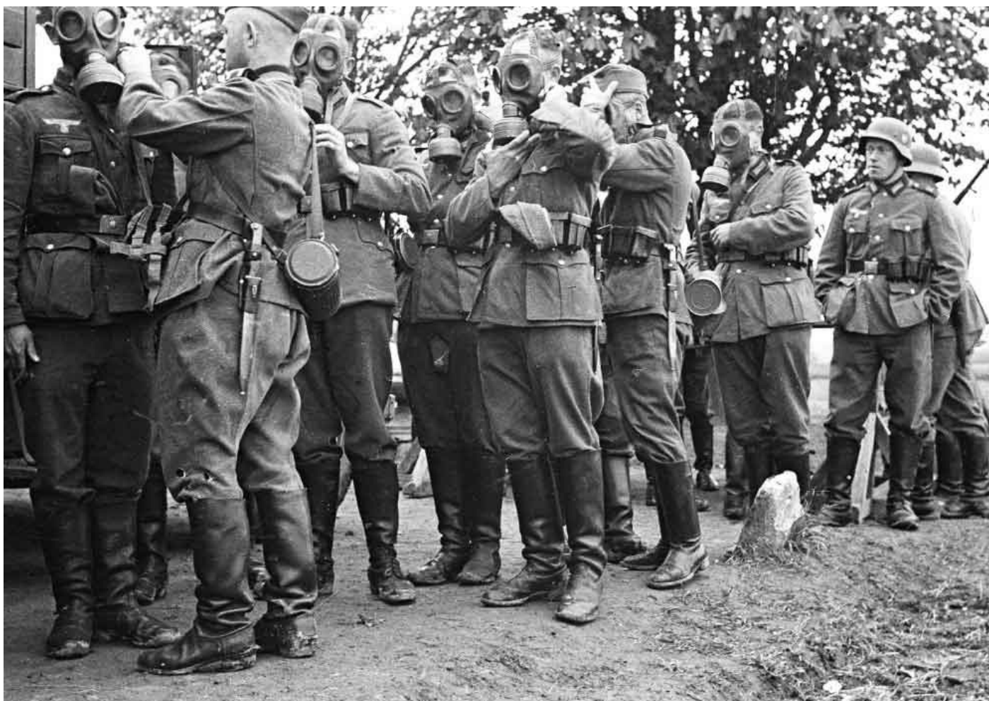
Recruits receive instructions on wearing the Gasmask 30 'S-Maske' . This rubberized canvas gas mask was manufactured in three sizes. Four different filters were issued: the Fe37, the Fe37 'R', the Fe41 and the Fe42. 'Fe'
