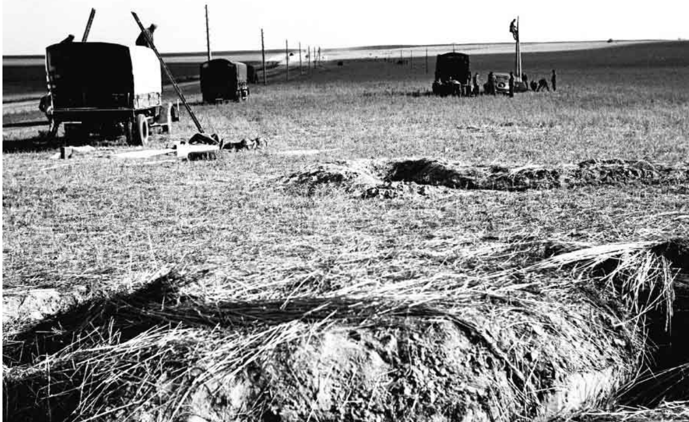
Drehkreuz telephone lines were generally erected fifty metres away from a road to prevent the poles being knocked down by vehicles. The inferior Soviet roads were usually wider than usual since drivers fought to dodge potholes and skirted churned-up areas. Note the trenches in the foreground.
