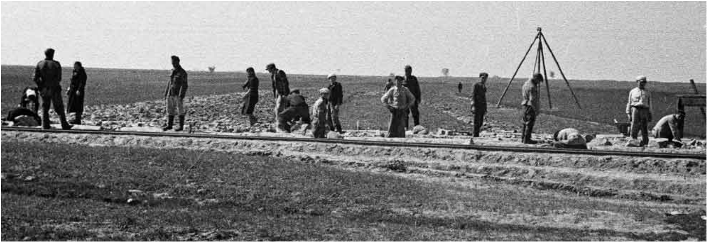
Building a road across the seemingly endless Ukrainian landscape.
