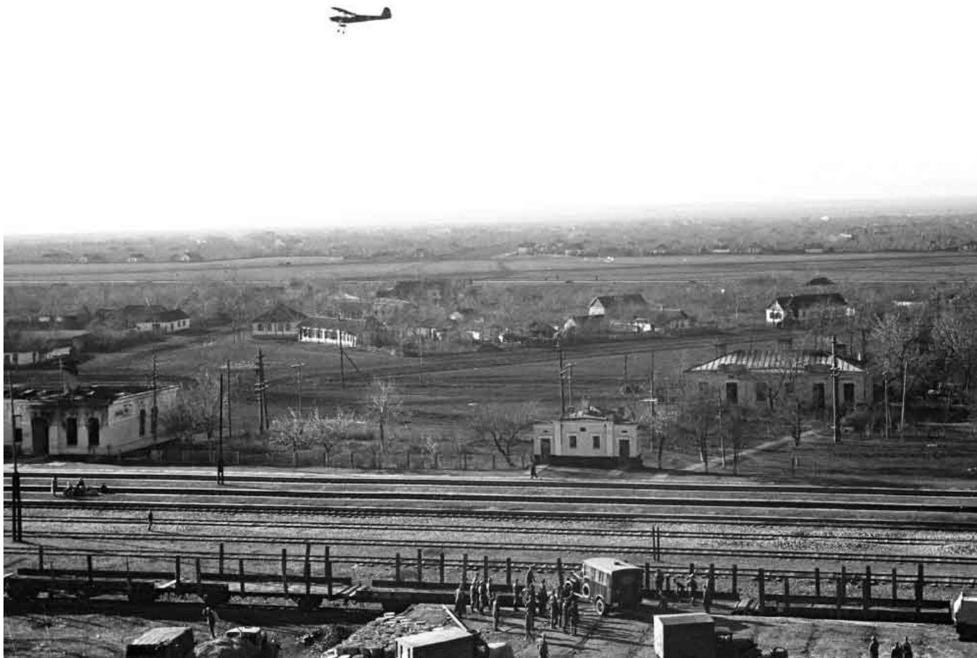
A Fieseler Fi 156 Storch liaison aircraft flies above flatbed railway carriages being loaded with vehicles. Soviet rail construction standards were inferior to those of Western Europe with lighter rails usually laid on a bed of sand, instead of rock and gravel. The wider distance between rail sleepers also precluded the use of heavy locomotives.
