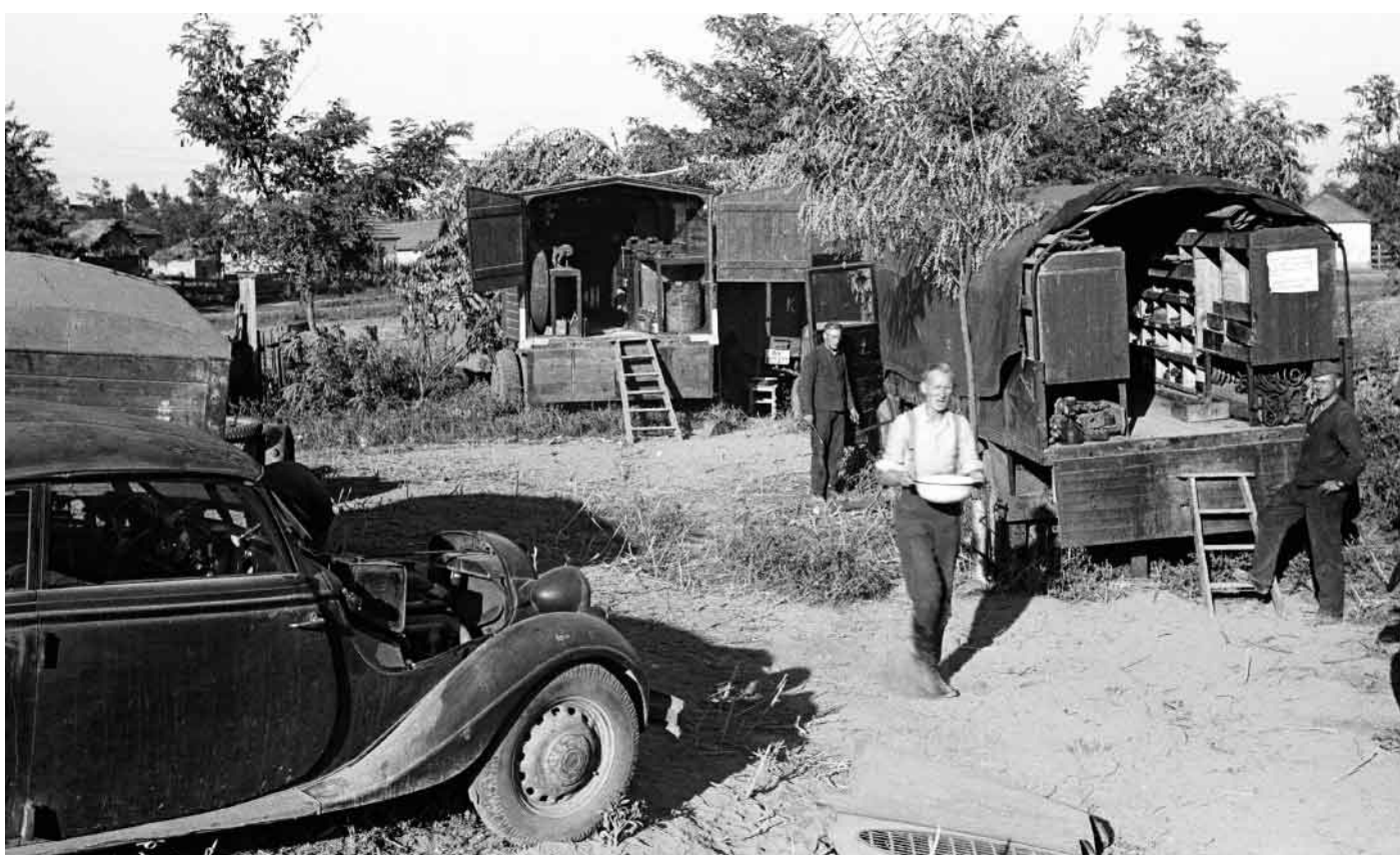
Machine-shop trucks contained equipment such as lathes, drilling machines and welding equipment. The vehicle on the right appears to be a Renault type AHN or AHR; the other vehicle is a field modification.
