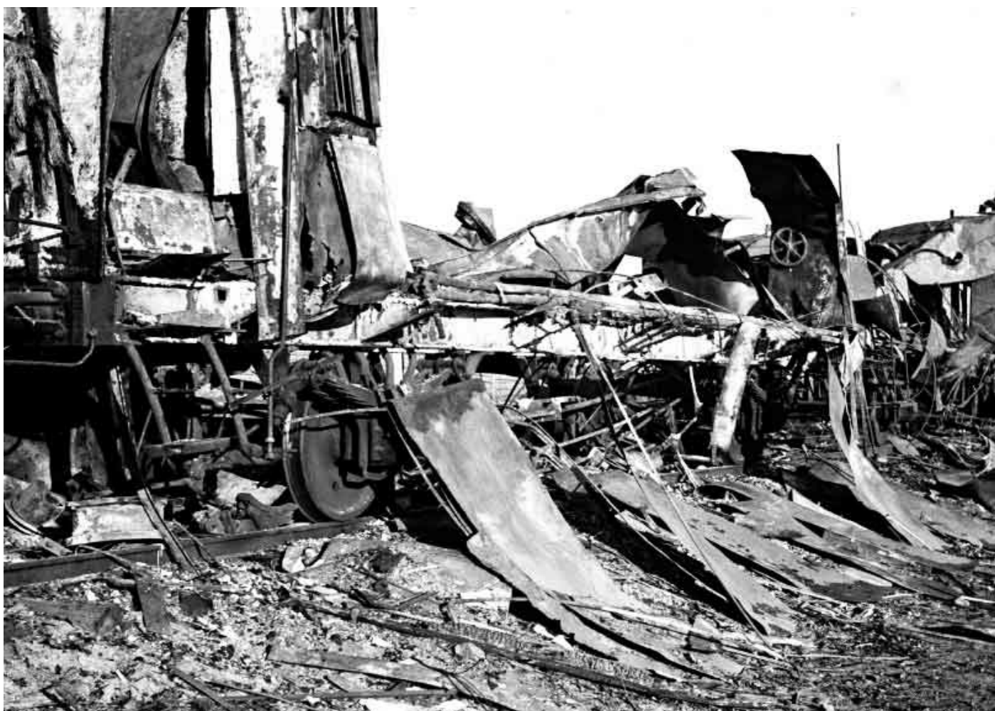
Top and above: Retreating Soviet troops systematically destroyed rolling stock, watering stations, switching yards and infrastructure associated with their railroad network. As Stalin urged in a radio broadcast on 3 July 1941: leave
