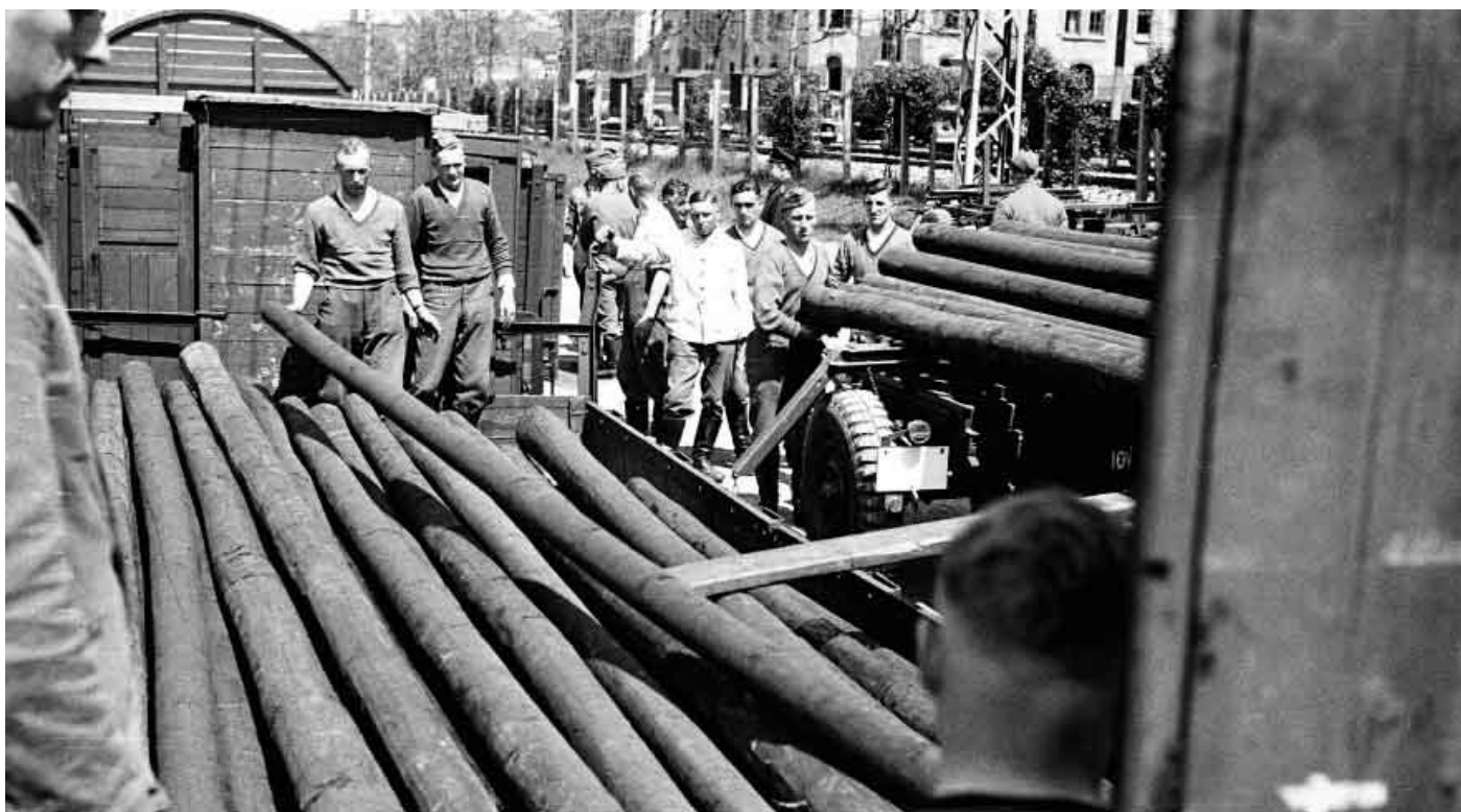
Top and above: Telegraph poles loaded onto a flatbed rail carriage from an Anhänger (1achs.) für Fernsprechbau (Sd.Ah. 21), a military trailer consisting of two identical single axle trailers coupled together. It had a carrying capacity of 3.7-tonnes.
