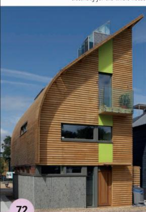
Triple-paned windows have The windcatcher three panes of glass with a channels air into layer of air between them. the house, providing The air stops heat from ventilation. The escaping, so you need less aluminum tubing energy to heat the house. reflects light inside. The "Lighthouse" is built with materials that absorb heat A biomass boiler burns wood during the day and pellets for heating and hot
