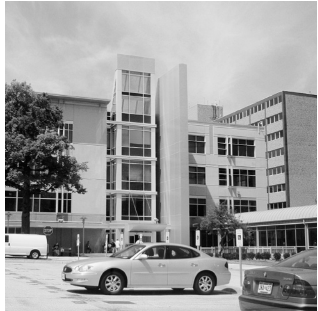
The headquarters of the Social Security Administration near Baltimore, Maryland. The Social Security Administration has more than 65,000 employees in 10 regional offices and nearly 1,400 field offices.
