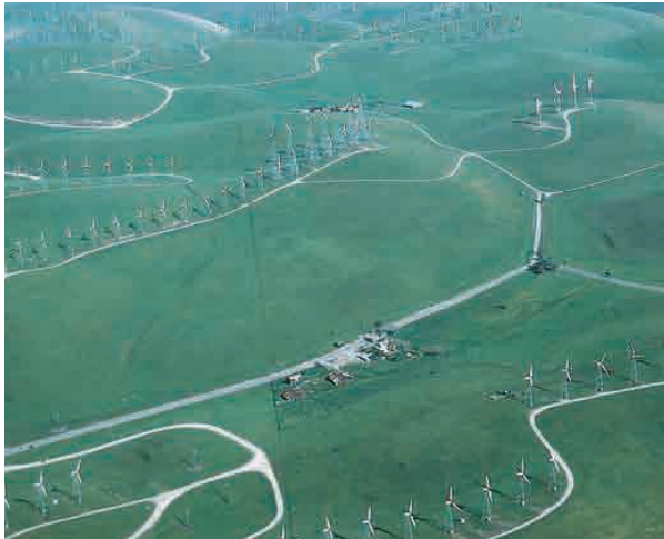
Tiverton, Ontario, wind generation station
