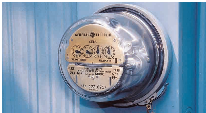
Figure 13.28 The electric meter in your home measures how much energy (in \text{kW} \cdot \text{h} ) that you use.
